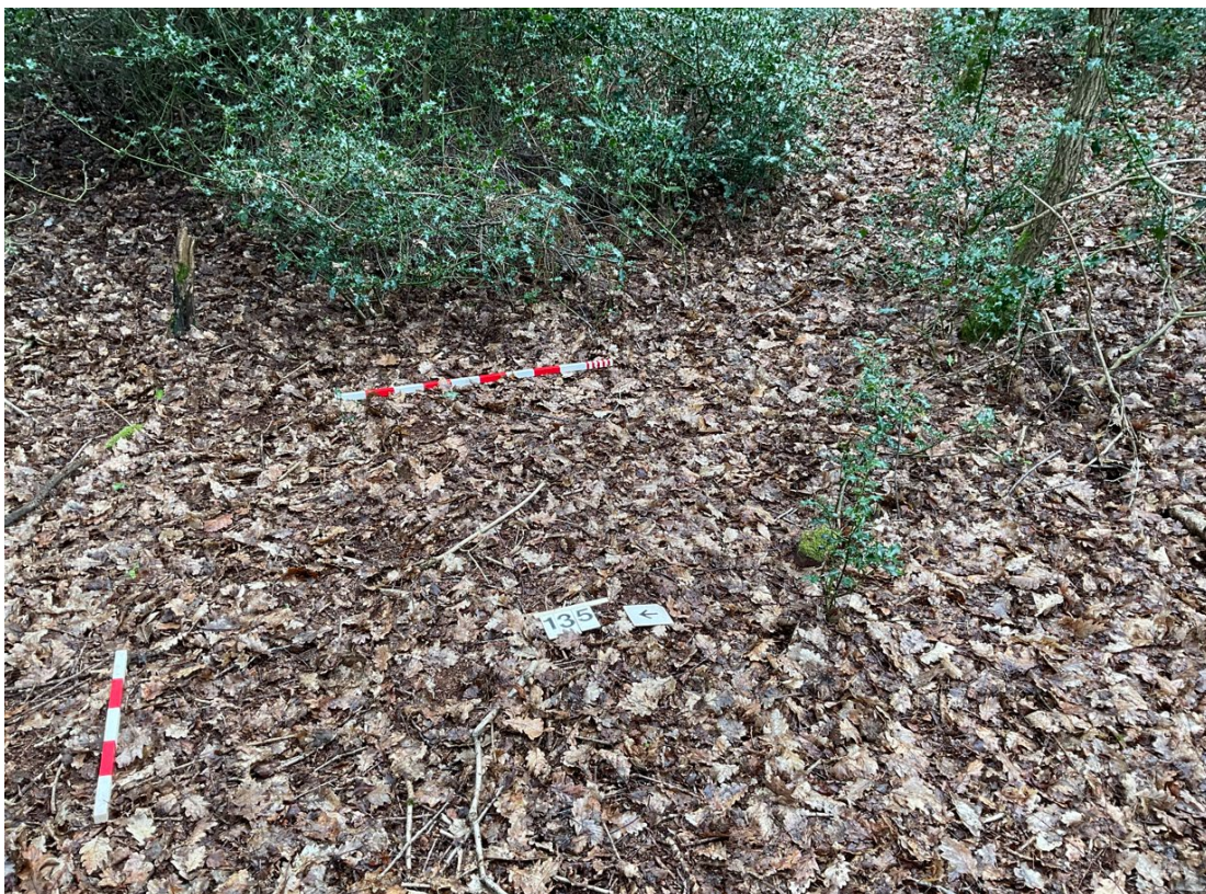
Figure 14: Roadside ditch surviving on west side of Agger within Streetly Wood (Photo 353, Feature Observation 135)
