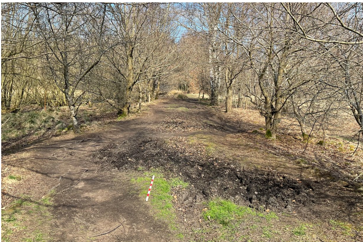
Figure 34: Feature Observation 167, Photo 475. Agger exposed by path erosion to the north of the railway
