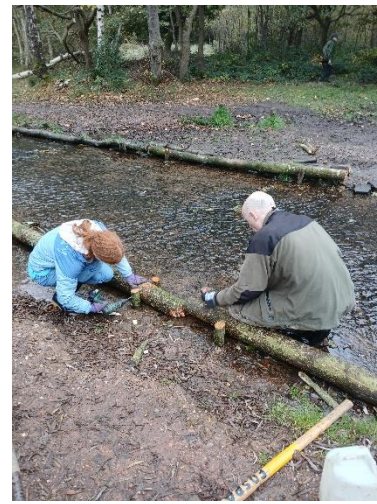
Replacing revetments
